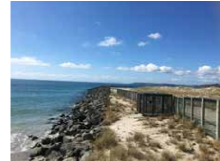
Groyne: Top - Storms on 20th April 2014 and just prior to lockdown on 15th March 2020
