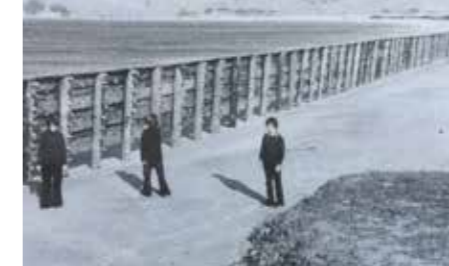
Erosion behind the wall
