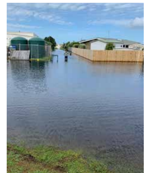
Flooding Darroch Reserve/Walkway 10, 15th February 2023
