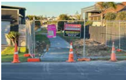
Concrete path repair and maintenance
